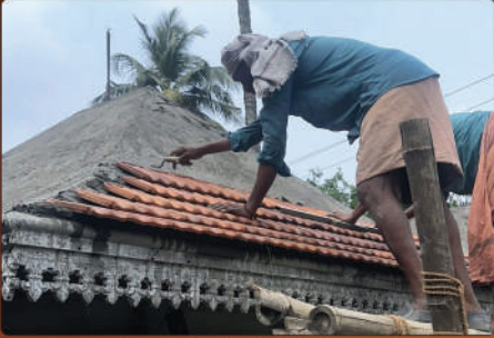
NINE UPADEVA FINISHING WORK
