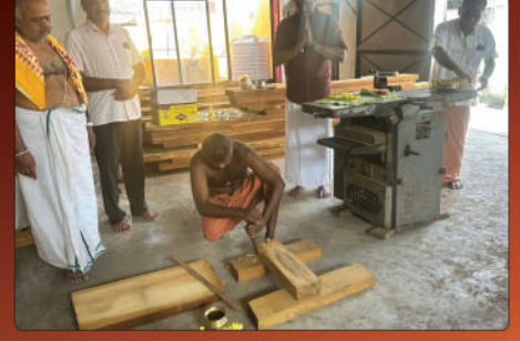
MAIN SANNIDHI WOOD WORK
