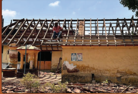
DEMOLISATION OF MAIN SANNIDHI
