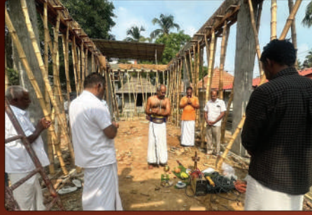
NADAPURA TRUSS WORK
